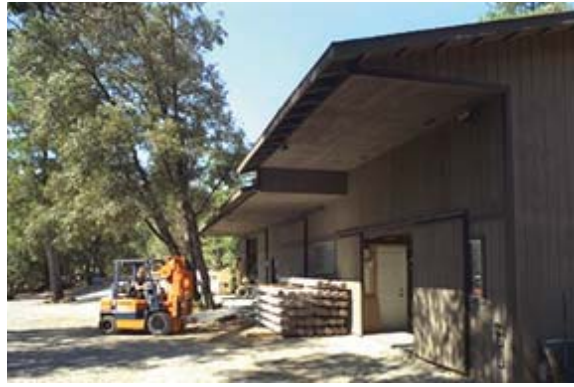
Modern, automated manufacturing & assembly facility
