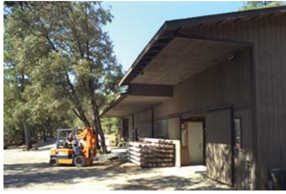
Modern, automated manufacturing & assembly facility
